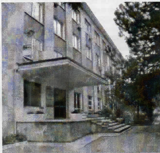
ISHP Tirane Lat 19°51.100' Long 41°20.754'
