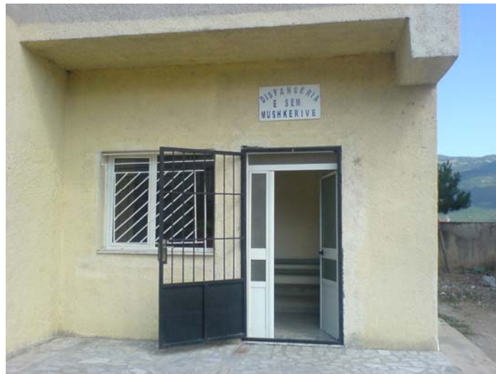
Reconstructed dispensary in Kukës
